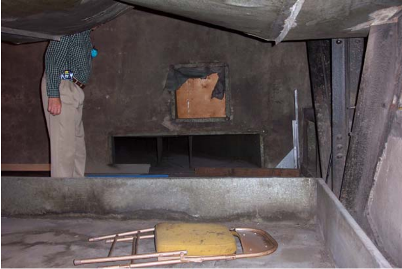
Fig 20 View inside return air plenum. Return air duct in back.
