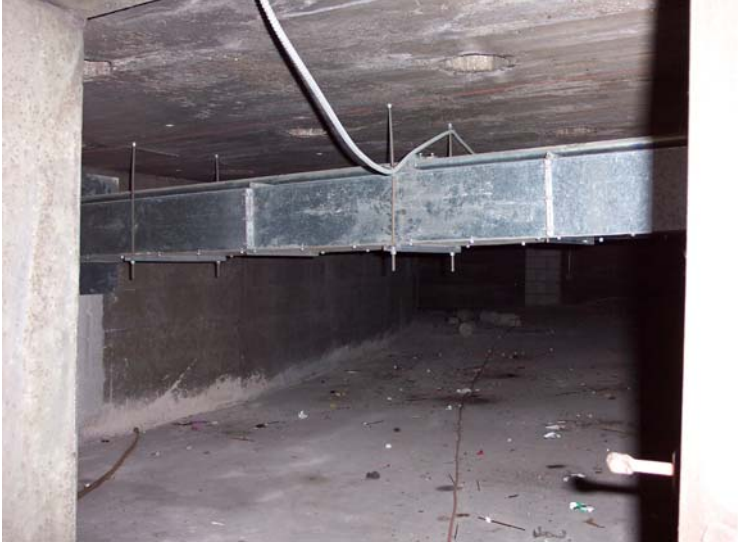
Fig 16B Another view inside main supply air plenum.
