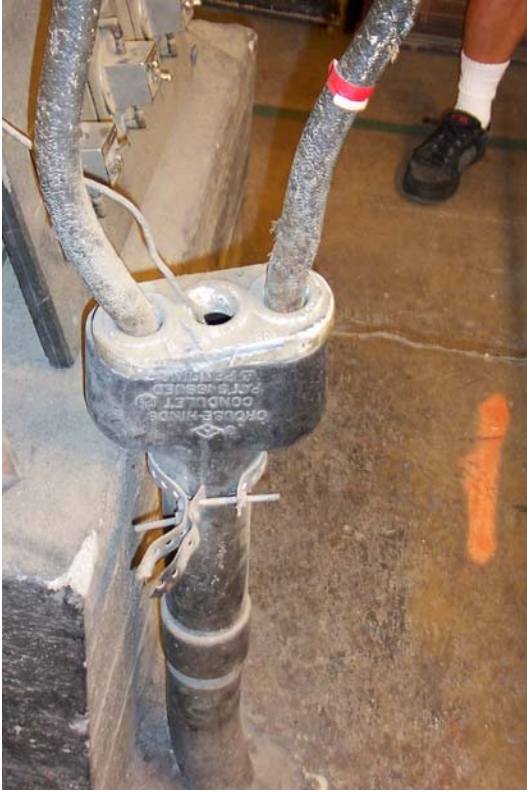
Fig 42 DC supply conduit and leads for compressor motor.
