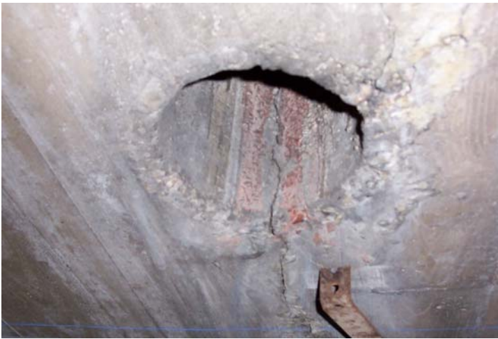
Fig 17 5 inch opening in supply plenum for mushroom ventilator.
