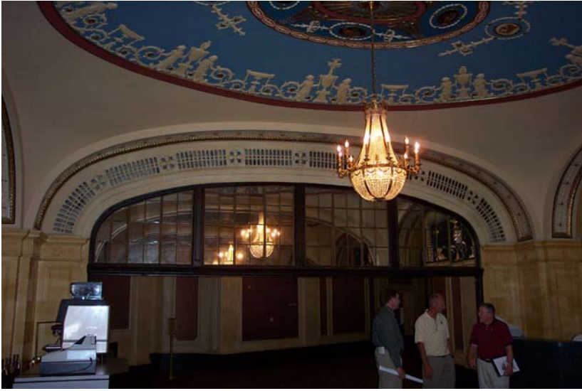
Fig 5 Lobby of Orpheum Theater. Note return air grilles above arch.
