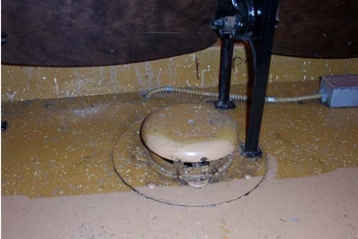
Fig 18 Mushroom ventilator for supply air under auditorium seats
