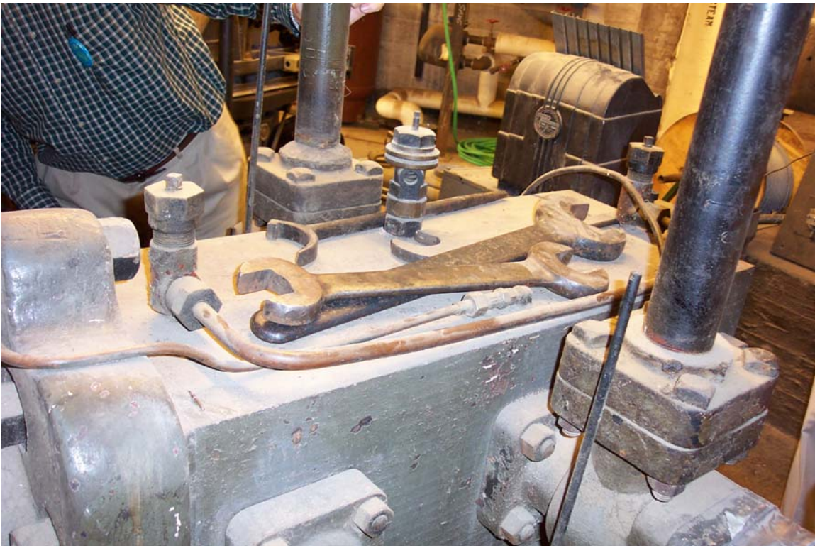
Fig 38 Close-up of compressor cylinder.
