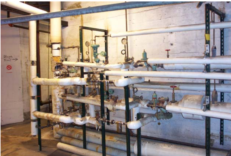
Fig 13 Steam reducing valves
