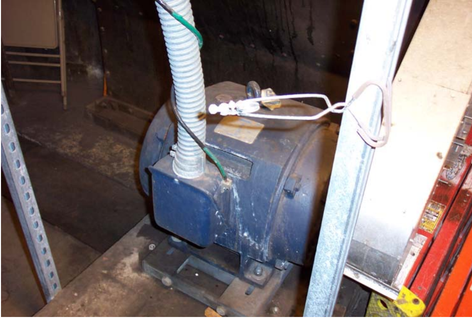
Fig 31 Return air fan 60 HP 3 phase AC motor installed in 1992.
