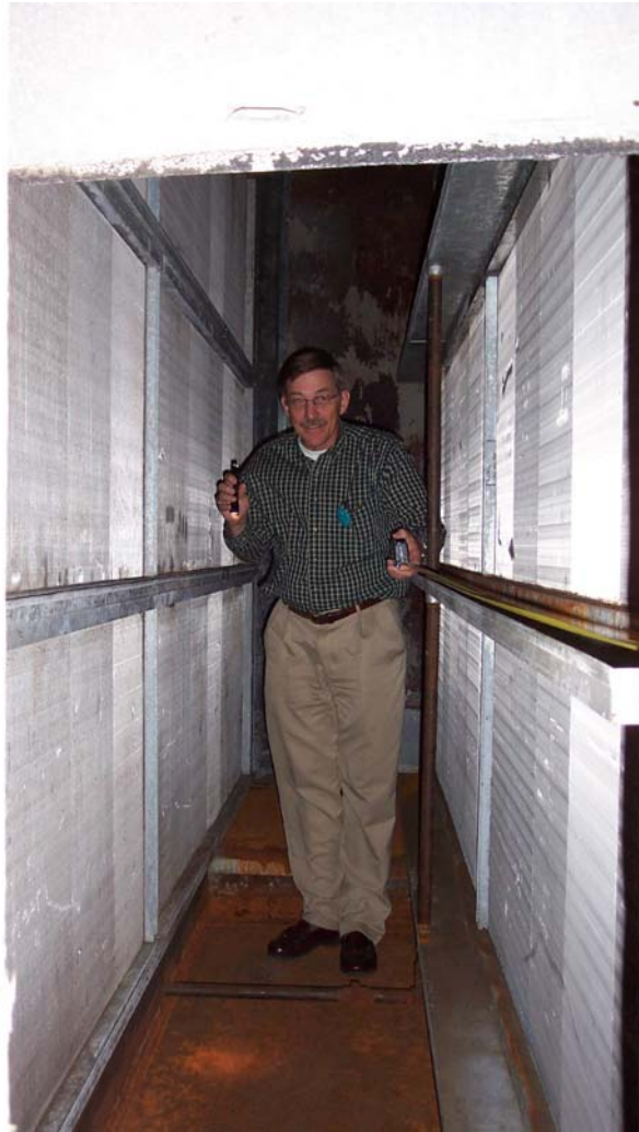
Figure 10 Rick Hermans between fin coils for heating and cooling, installed in 1988.
