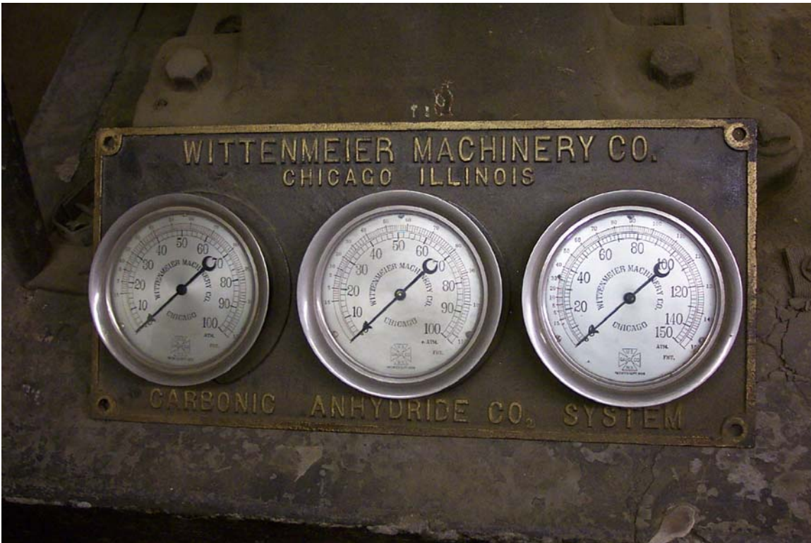
Fig 40 Compressor gauge board.
