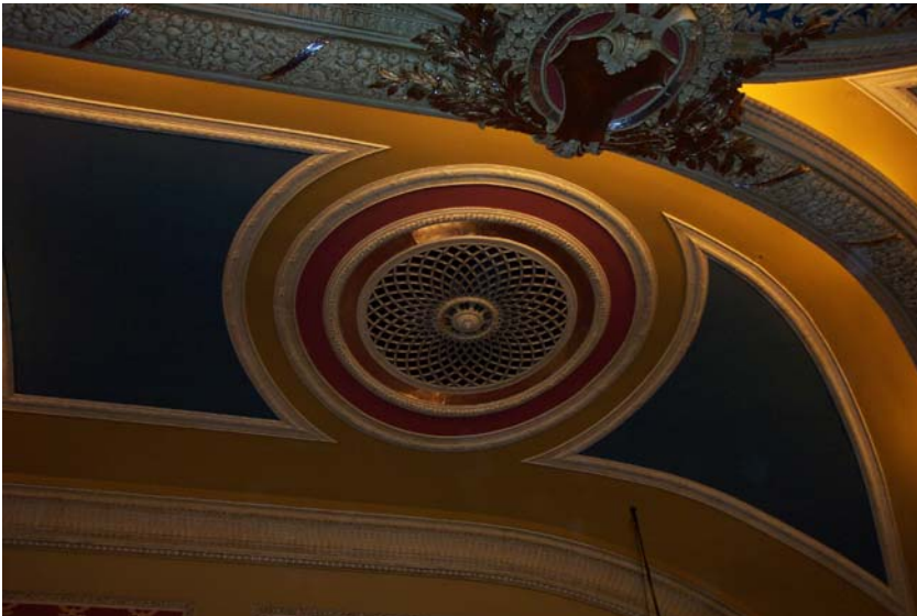
Fig 19 Return air grille in auditorium ceiling
