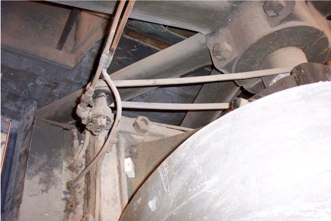
Fig 39 Flywheel bearing area showing oil pump for bearings.
