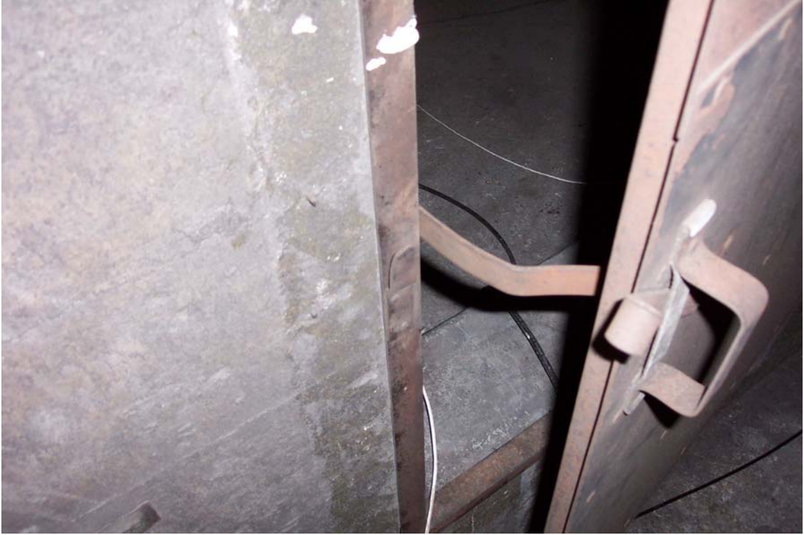
Fig 45 Supply air damper with adjustable door latch for balancing air to individual supply ducts.
