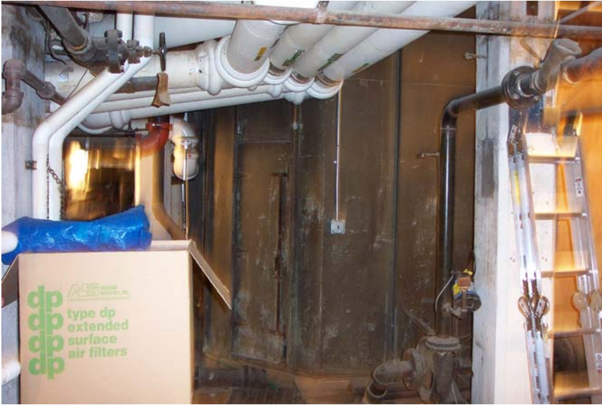
Fig 14 Chilled water pipes (overhead) from downtown district system
