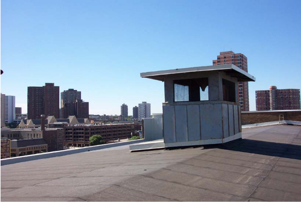
Fig 24 Exhaust air turret on roof.
