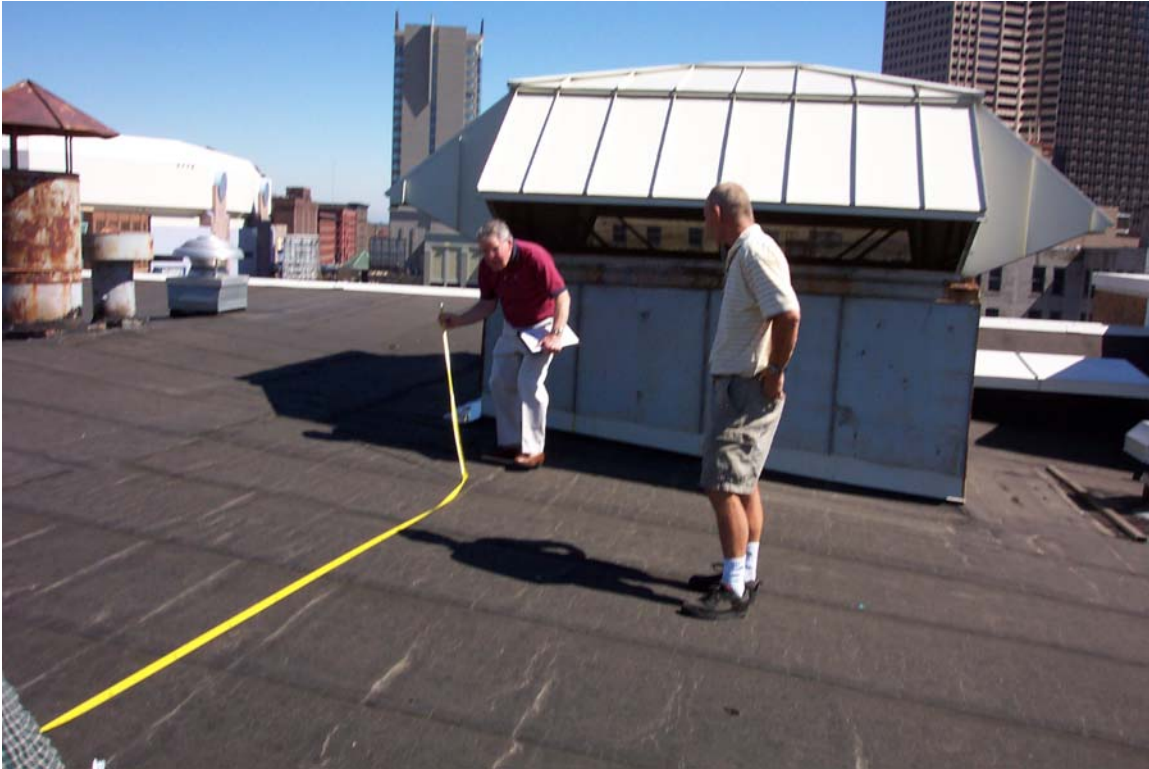
Fig 22 Fresh air inlet on roof.
