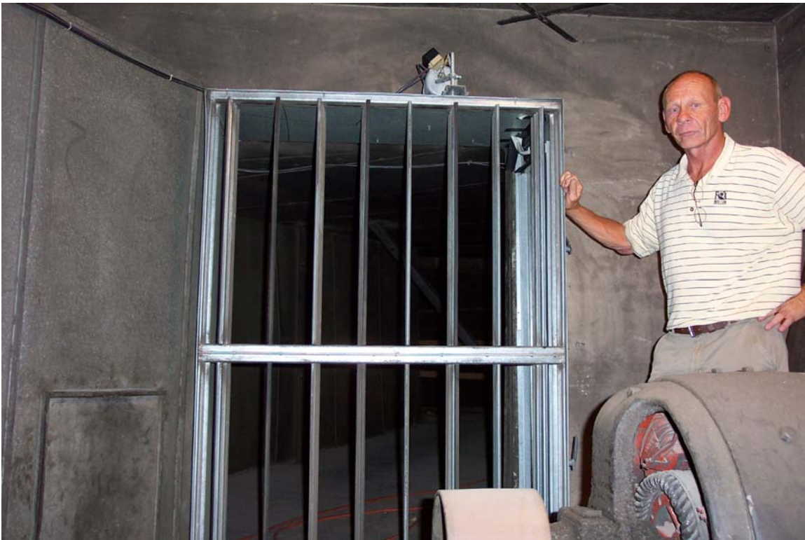
Fig 23 Fresh air inlet dampers in return air plenum. Old DC fan motor in foreground.
