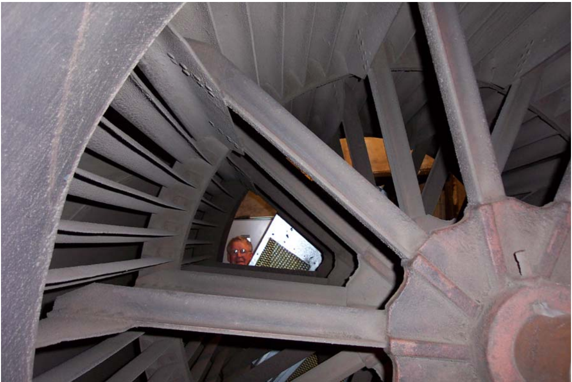
Fig 27 Bill Murray looking through return air fan cage.
