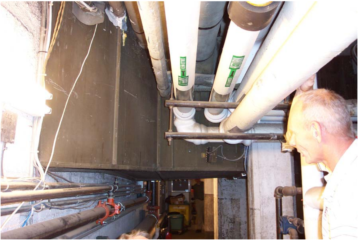
Fig 29 Dave Marietta looking at original steel supply duct.
