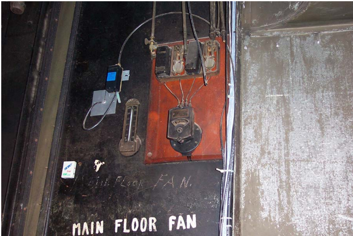
Fig 34 Johnson 4 stage controls for main supply air.
