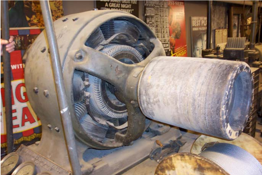
Fig 9 100 HP DC motor for CO2 Compressor.
