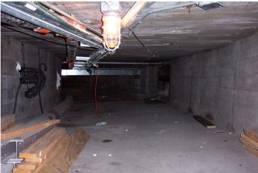
Fig 16A View inside main supply air plenum.
