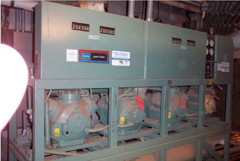
Fig 12 Carrier 120 HP Chiller installed in 1988
