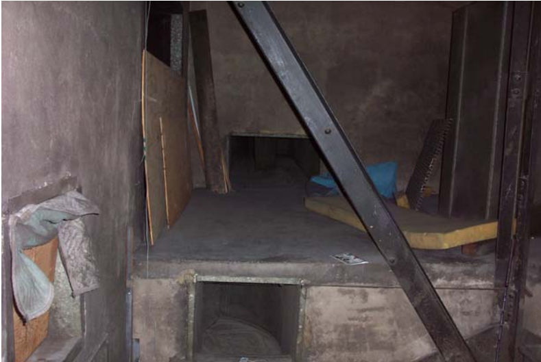
Fig 21 View inside return air plenum showing return air ducts.
