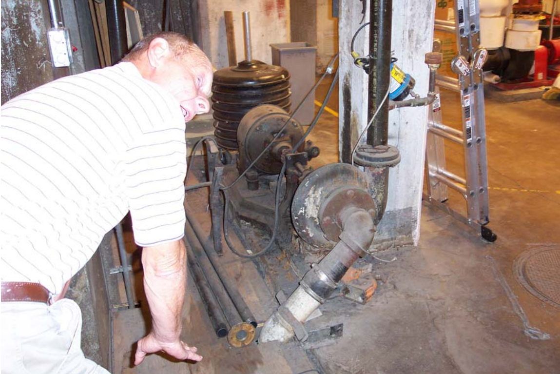
Fig 32 DC motor driven pump for air washer
